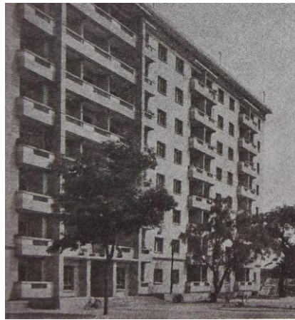
Figure 5. Unknown. Fusuijing Building. Date unknown.
