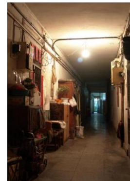
Figure 8. Unknown. Corridor of the Fusuijing Building , 2016. Photograph. Obtained from Yi Fu
