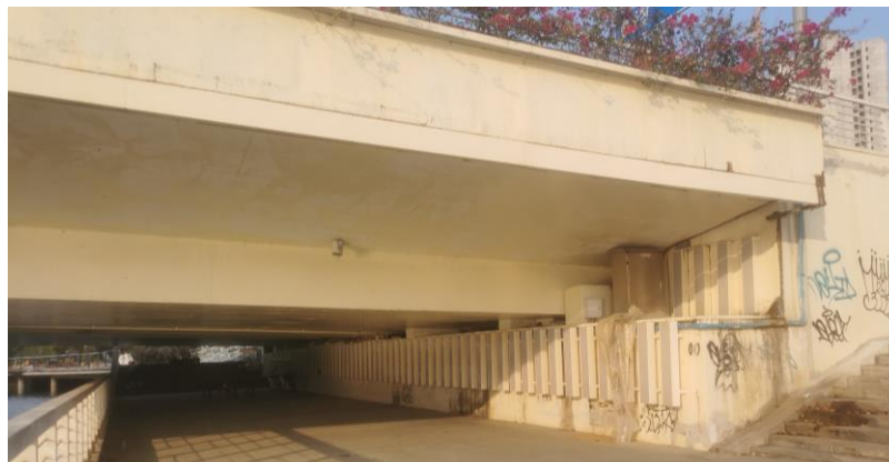
Figure 1. Current situation of underpass space of municipal bridge
