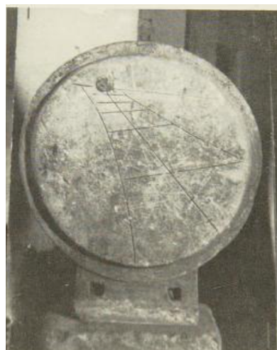
Figure 7. Meridian sundial. Gibbs, Plate 60, p. 367 [8]
