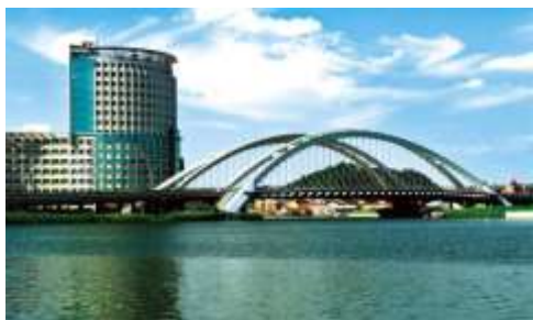
Figure 3. The Yufeng Bridge.
