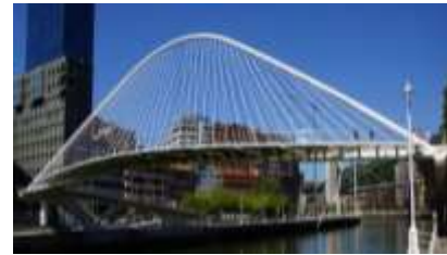
Figure 8. The Campo Volantin Footbridge.
