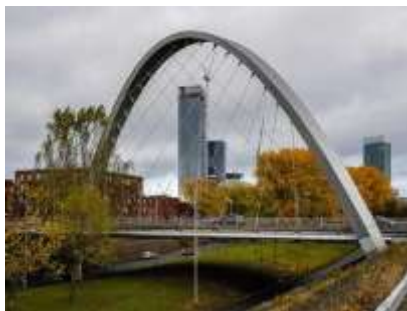
Figure 13. The Hulme arch bridge.
